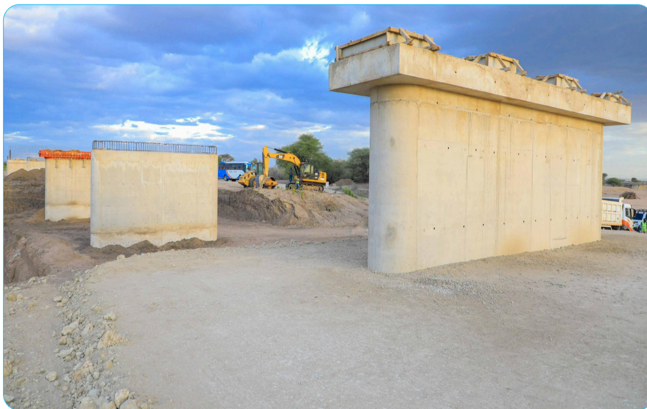
Itembe Bridge under construction (Photo: Ministry of Works)
